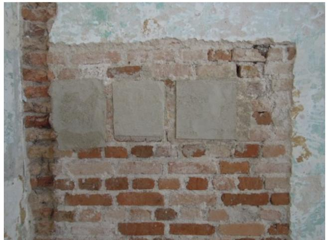
*Trial lime mortar samples on historic brickwork*
